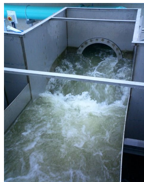
View of the submerged weir
