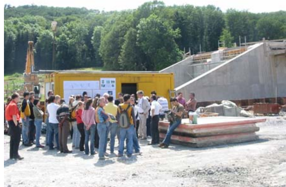
Participants getting technical explanations in front of the outlet structure
