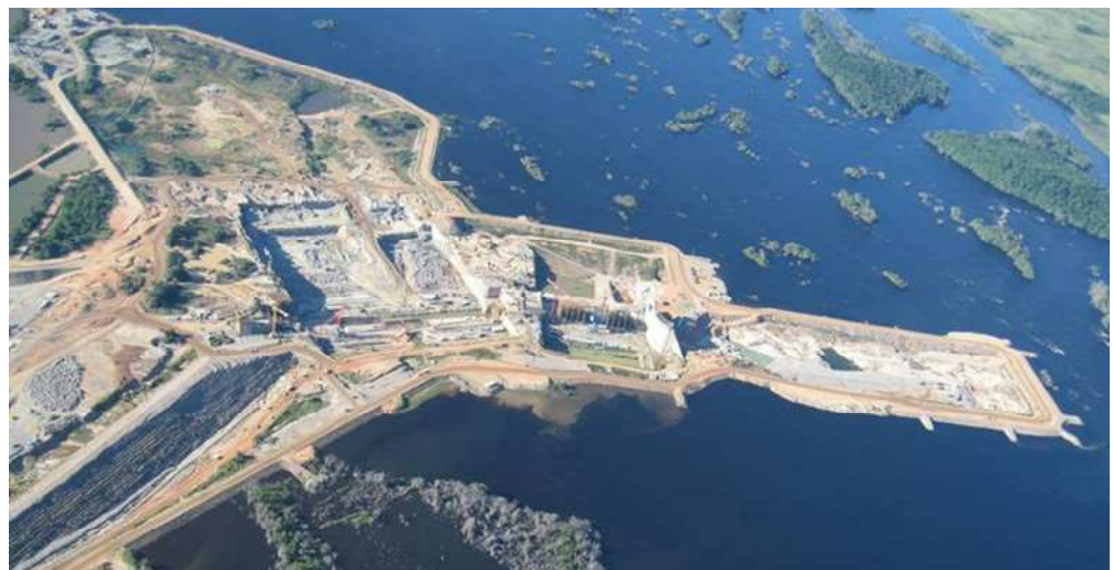
Tocoma Project-First Stage of River Diversion (Oct 2008)
